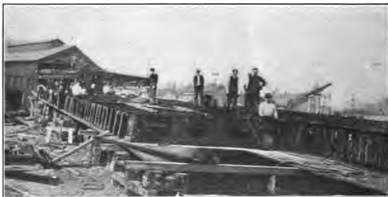
FIG. 83.—Portion of double bottom framing completely erected.
