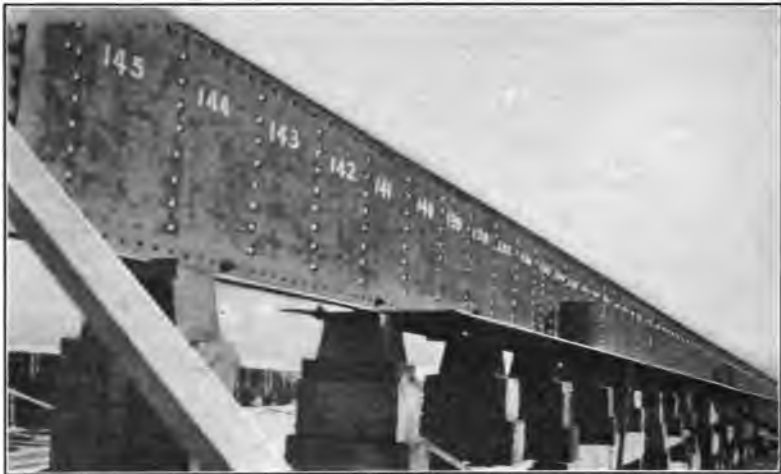
FIG. 80.—Flat and centre vertical keel plates in place on blocks.
