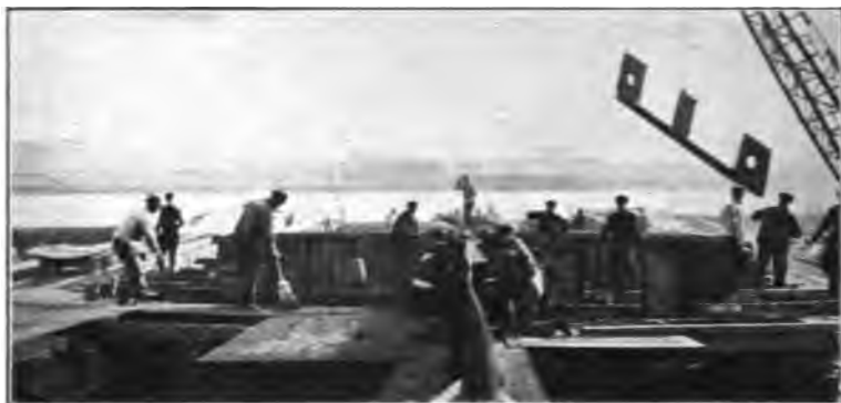
FIG. 82.—Erecting double bottom framing.
